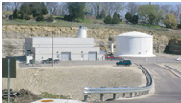
Herculaneum Water Treatment Plant
