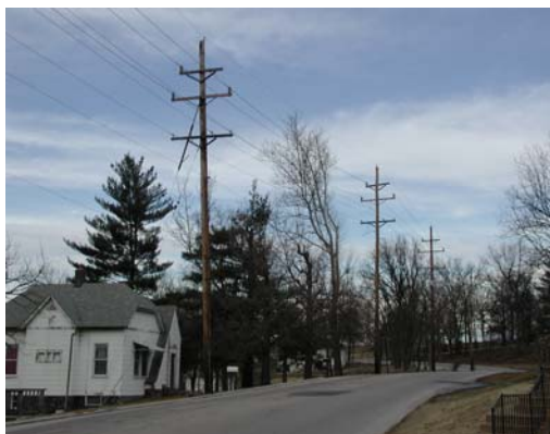
Electric Lines Over the City
