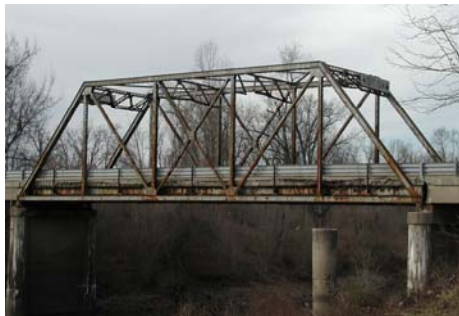
Joachim Creek Bridge
