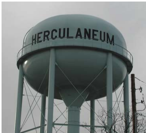
Herculaneum Water Tower
